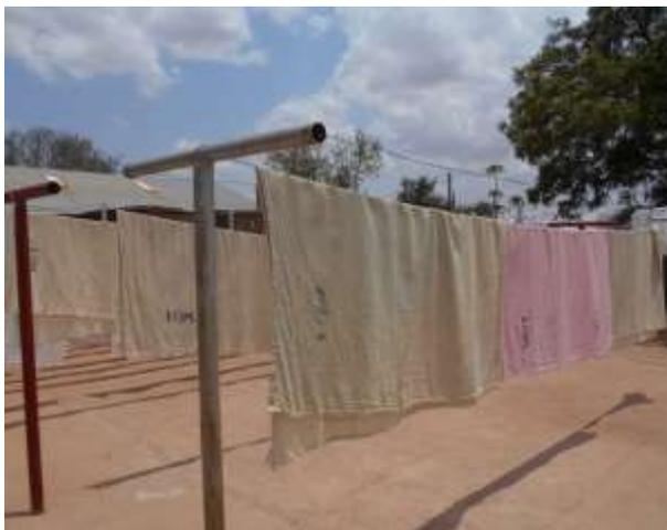
The hospital laundry drying area had a soil floor, which soon turned to mud from the dripping washing. Also there were too few poles and drying lines. A stone + concrete floor and additional poles have been put in.
